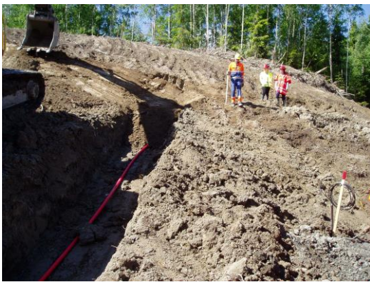
Figure 1 Installation of conduit for settlement
